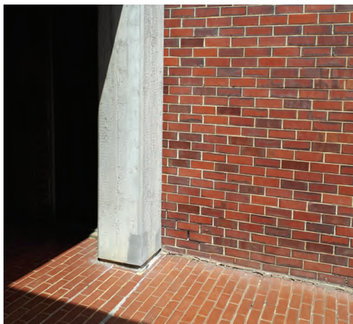
Image 9. A palette of 'Distinctly Curtin' materials at the T.L. Robertson library; formboard concrete and mortared red brick laid in a stretcher bond style. Source: UDLA.
