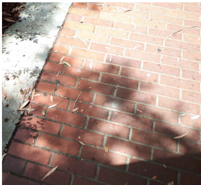
Image 8. Existing mortared red brick, laid in a stretcher bond with a concrete edge located on western side of B103. Source: UDLA.
