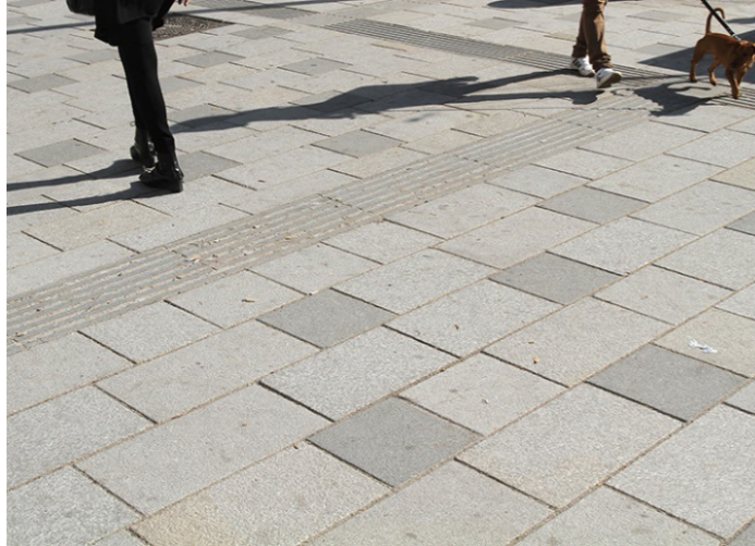
Figure 9: Mariahilfer Straße, Vienna (left) – Directional tactiles designating the safe route along the pedestrian sidewalk.
