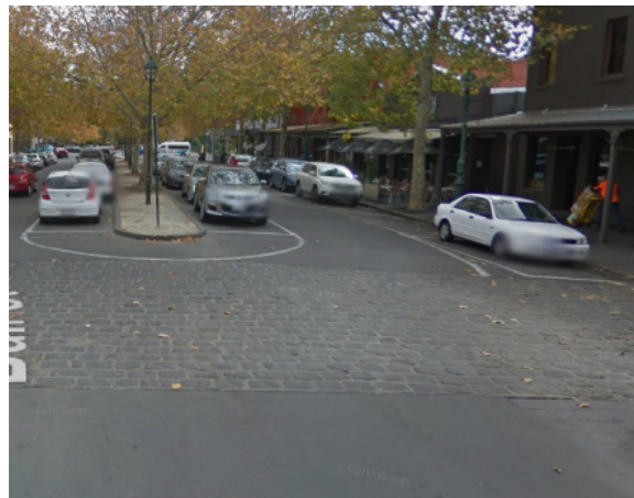
Figure 13: An example of a textured pavement rumble strip is an effective traffic control technique within the transition zone of a shared zone.
