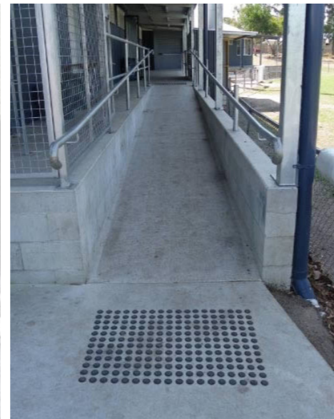
Figure 11: Stainless Steel Tactiles (left) – Tactile Indicators provides stainless steel tactiles to be used at pedestrian crossings in shared zones. Tactiles are drilled and glued with a 12mm stem (5-year warranty). Black PVC dot Tactiles (right) – where stainless tactiles do not meet the 30% luminance contrast, black tactiles should be used.
