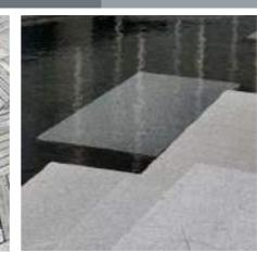
Element: timber decking Indicative Material: hardwood Element: intermediate terraces/ steps Indicative Material: in situ concrete, light grey to charcoal grey, textured finishes
