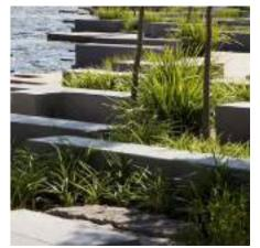
Element: stepping stones/seating blocks to lower terraces Indicative Material: exposed aggregate concrete/ rough hewn stone
