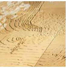
Element: main promenade and terracing Indicative Material: in situ concrete/exposed aggregate concrete Colour: light beige to ochre
