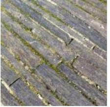
Element: feature paving off main promenade Indicative Material: exposed aggregate concrete/granite strip
